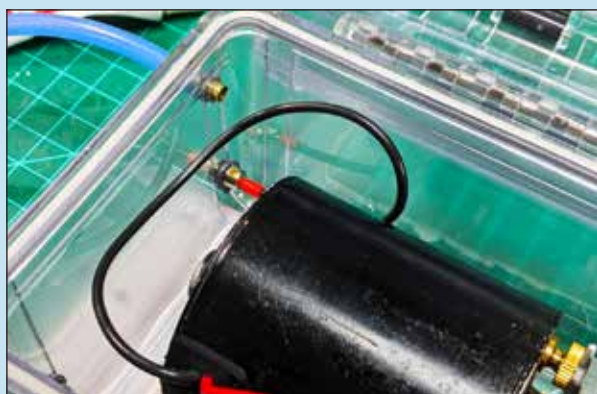
Fig. 25: Internal electrical connections.
